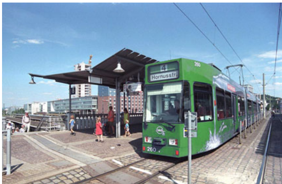
Terminal over Freiburg banegård
